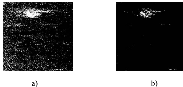
Figure 7. Image of the pavement damage: a) 10% of significant coefficients, b) 1% of significant coefficients
