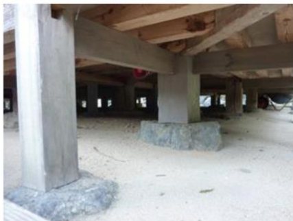
Photo 2 Post erected on a foundation stone
