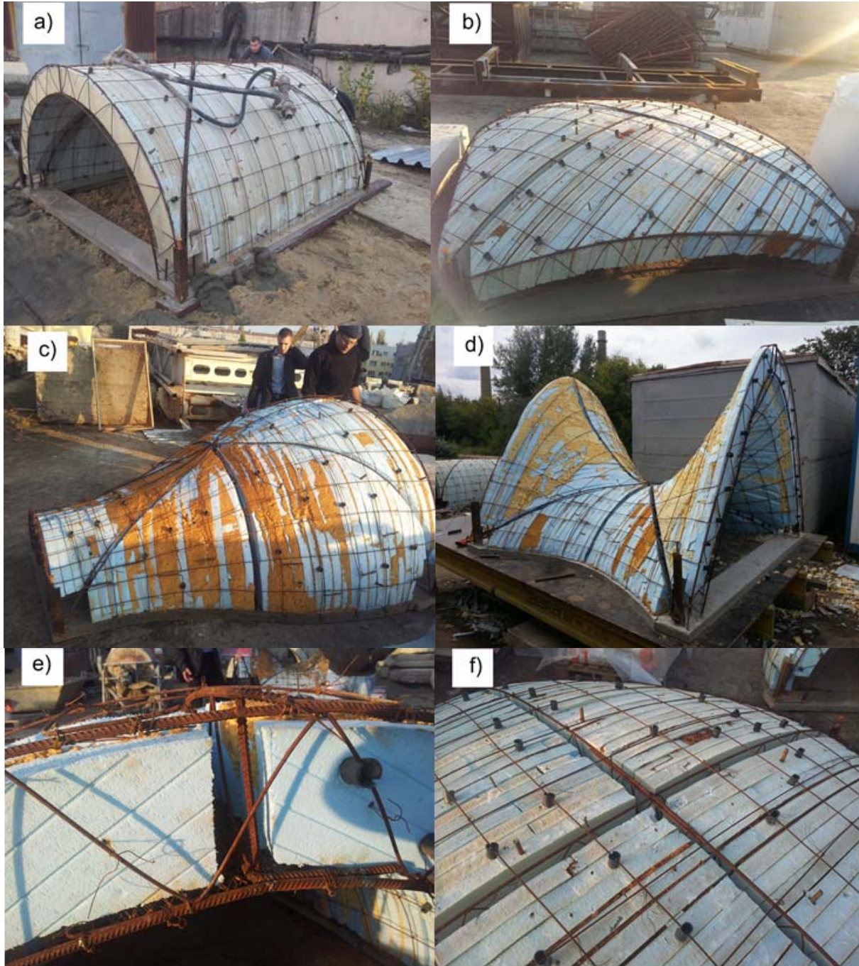
Fig.9 Self-bearing frames for concreting of reinforced concrete shells: a) frame for cylinder; b) frame for sphere; c) frame for nodoid; d) frame for hyperboloid; e) view of flat skeleton fragment; f) arrangement of inserts within self-bearing frame
