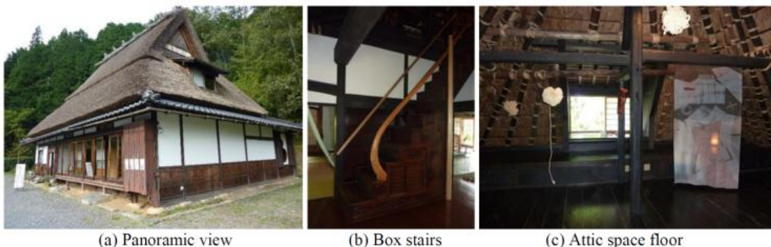
Photo 1. One-storey thatched roof wooden structure
