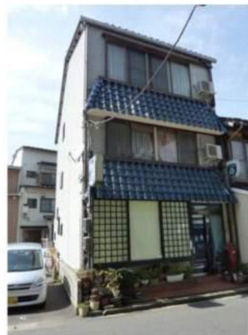
Photo 1 Elevation view of 3-story wooden house
