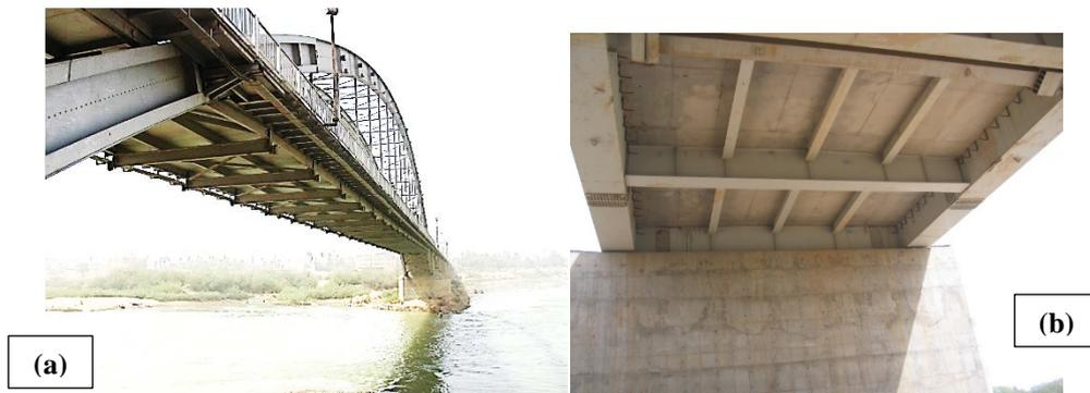
**Figure 1.** Typical bridge superstructures with transverse floor beams; (a) Steel arch bridge, (b) Steel box girder bridge
