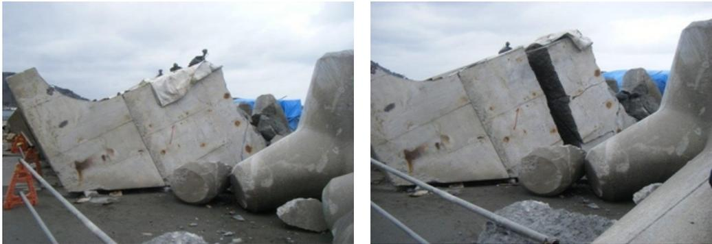
Figure 1. Cracking construction of an unnecessary concrete caisson by SPC.
