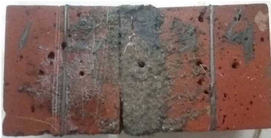
Fig 3. Mortar plus bricks system were cut into 5 segments
