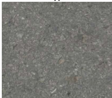
Fig.5 (a) Core sample 3 original pavement
