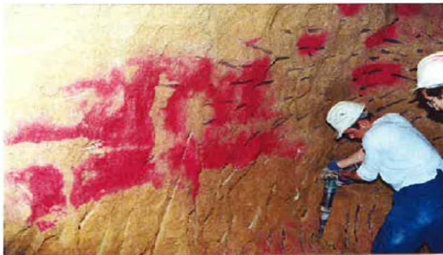
Figure 10. Ease of excavation due to grouting (pink in color) carried out prior to excavation
