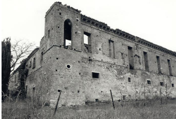
Figure 6: South-West tower of the Friary
