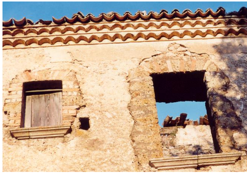
Figure 18: Limestone thresholds existing on the west prospect
